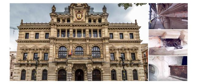
At the beginning of spring 2000 while working on the rehabilitation of the elegant Regional Palace owned by the Bizkaia Regional Deputation, CONSTRUCCIONES AMENABAR encountered broken lintels, deformed cornices and deteriorated, out of plumb, pinnacles on the last floor of the building.
